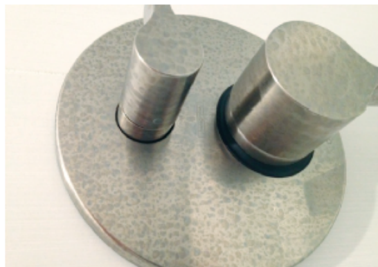
Figure 3. Silica deposits on a polished chrome shower fixture
